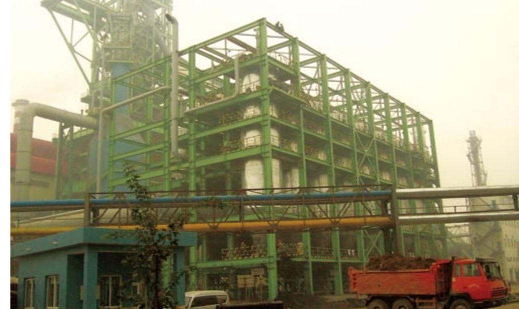
济钢3号1750m 3 高炉煤气干法除尘系统总承包工程 General contract project for BFG dry dedusting system for Jigang's 3# 1750m 3 BF
