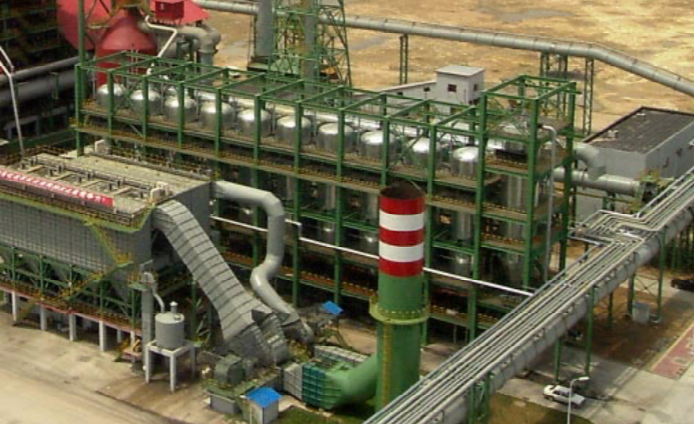
首秦1号1200m 3 高炉煤气干法除尘系统总承包工程 General contract project for BFG dry dedusting system for Shouqin's 1# 1200m 3 BF
