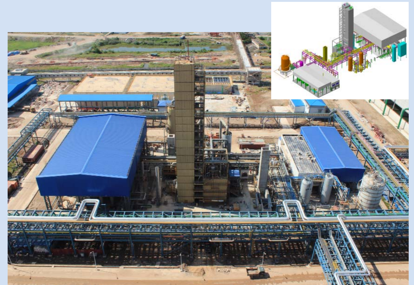
正在建设中的越南（煤头）化肥项目 35000m 3 /h 制氧工程 Vietnam Ninh Binh Fine Coal Based Urea Plant project 35000m 3 /h air separation project is under construction.
